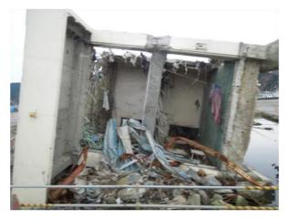
Picture 7: Disaster debris generated by building collapse (Onagawa)
