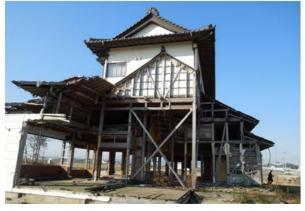
Picture 11: Remained house whose ground floor was washed away by the tsunami
